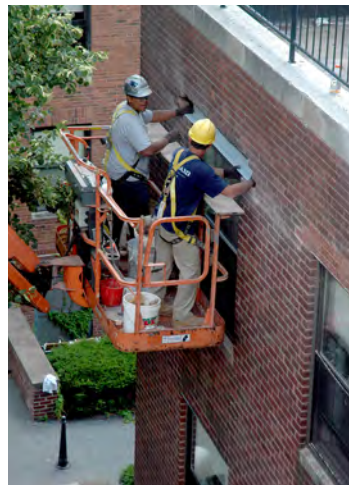
Window and Lintel repairs
